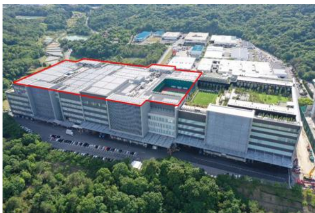
Solar power generation system at Kuwabata Plant
